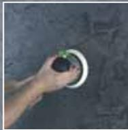
4. The surface is then polished with a grinding disc with an abrasive grain size of 120.
