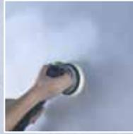
5. After approx. 4 – 5 hours the surface is polished with a suitable eccentric grinder using a grinding disc with an abrasive grain size of 120.
