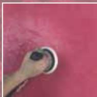
3. After approx. 4 – 5 hours the sharp points are broken with a suitable eccentric grinder using a grinding disc with an abrasive grain size of 80.
