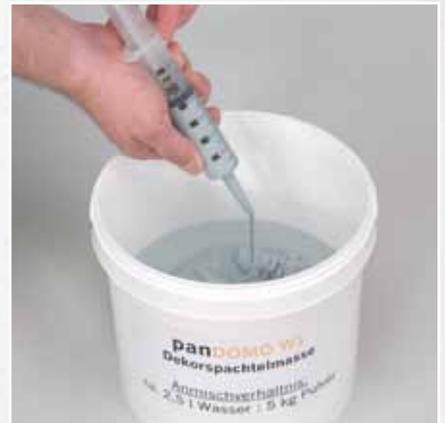
2. From the sprayer the measured quantity of colour is added to the mixing water.
