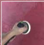
5. After approx. 3 – 4 hours the surface is polished with an eccentric grinder using a grinding disc with an abrasive grain size of 120.
